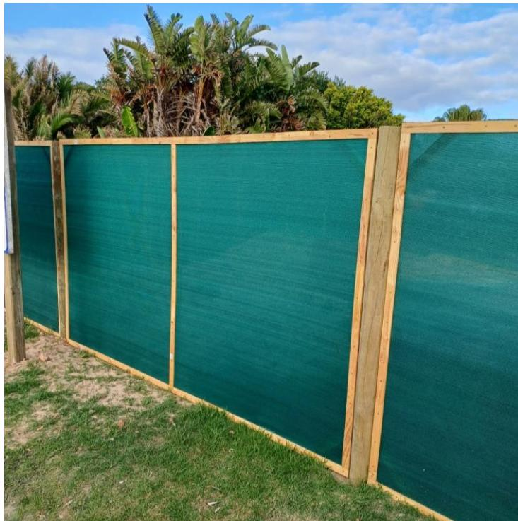
The upright steel/wooden supports need to be kept spirit level straight with the shade cloth pulled tight. These support poles may not be installed to the outside of the screening.
